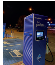
Charging is available at more and more gas stations.
